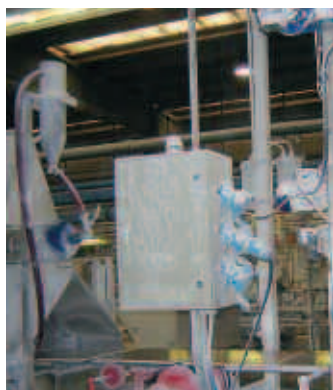
The DSN Series NEMA 4X protection and the DS Series 3R protection is achieved simply by mating the plug and receptacle
