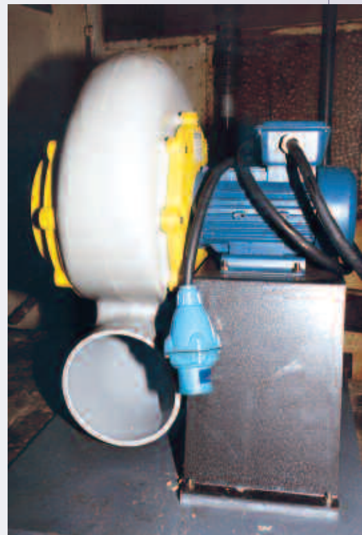
Decontactors enable equipment to be connected and disconnected with plug & play simplicity.
