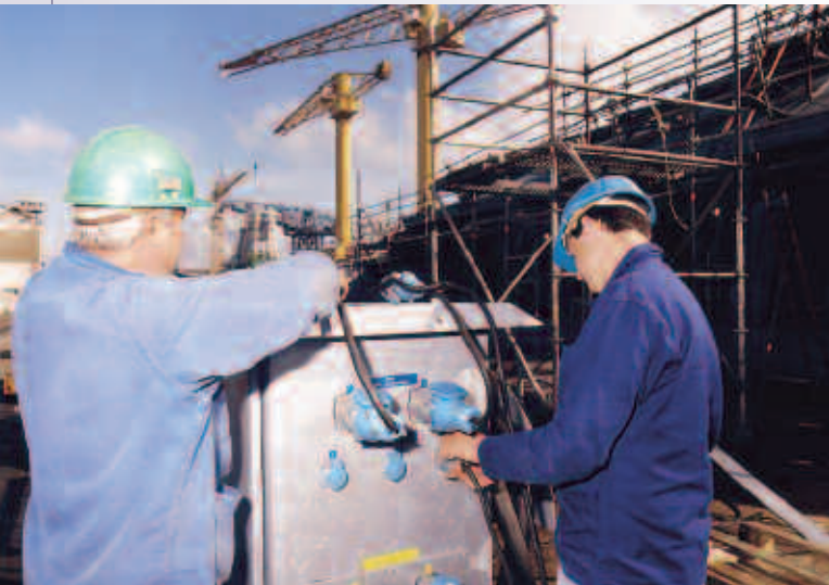
Pressing the pawl on the DECONTACTOR receptacle safely ejects the plug to its rest (OFF) position
